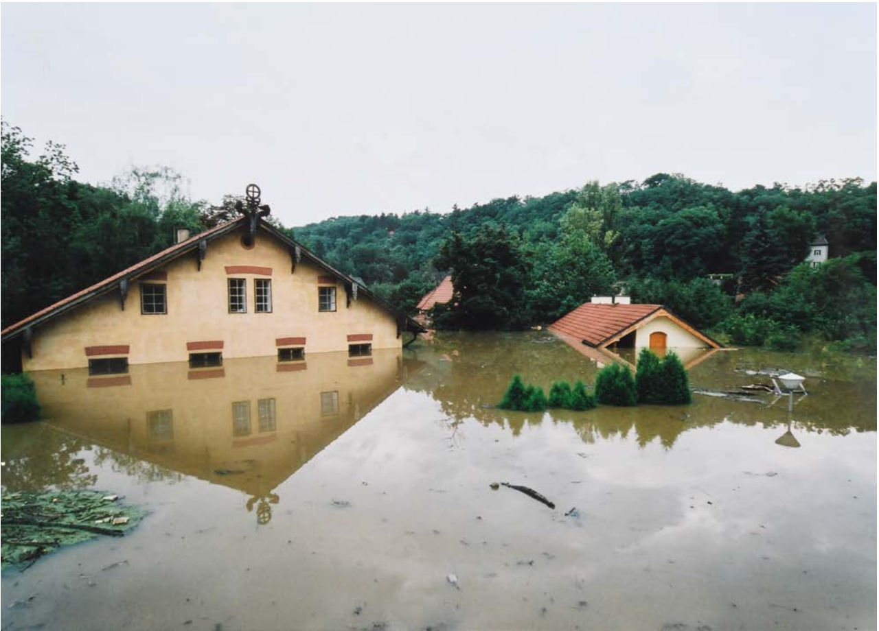
The floods in 2002, the flooded buildings of Central Bohemian Museum in Roztoky near Prague
