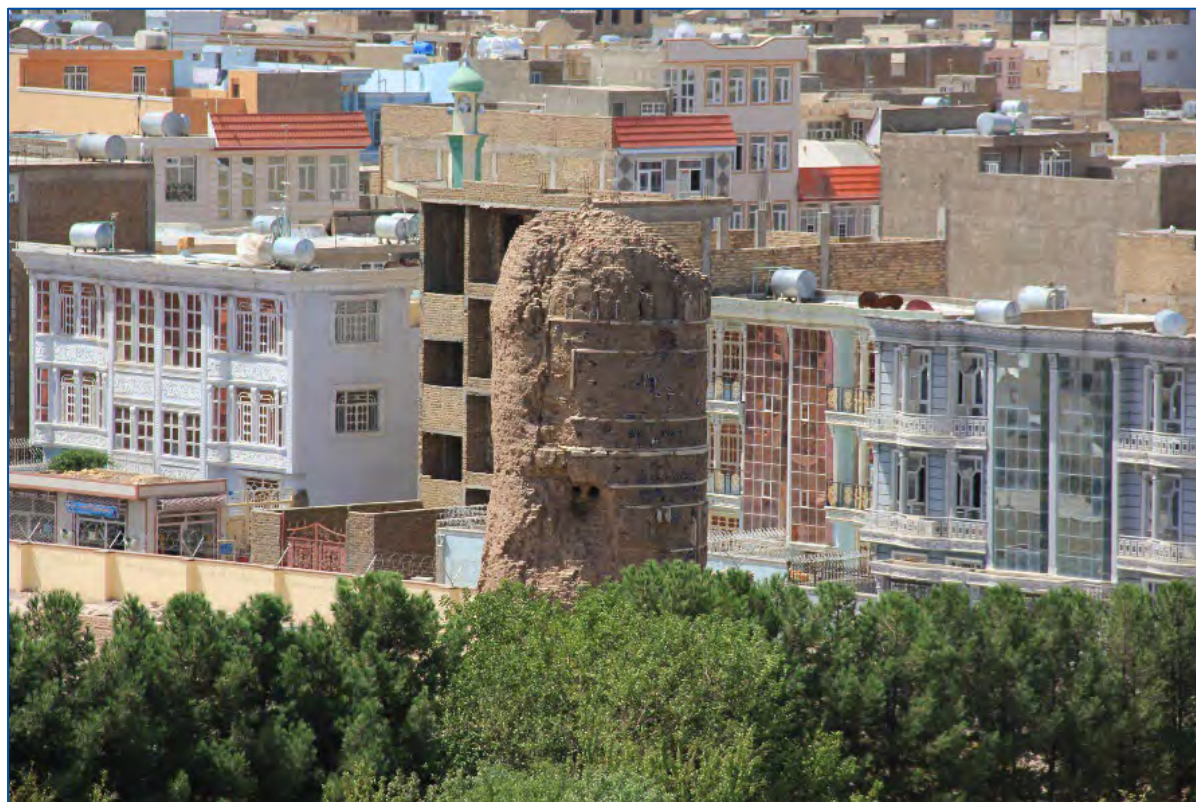
Figure 6: Current condition of the only remaining minaret of the Gohar Shad Mosque, collapsed by the bombing of Russian planes, 2016 © Author.
