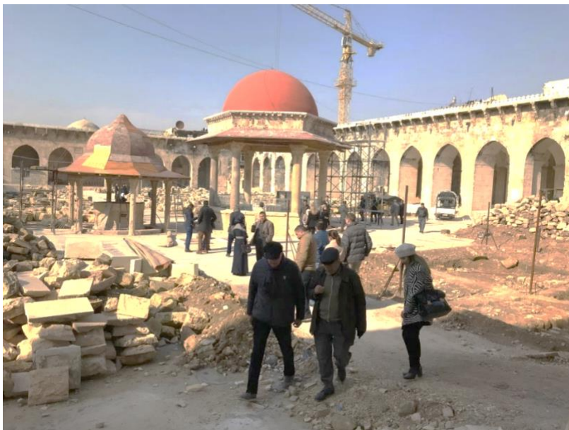
Figure 25: On-site inspection of the damaged Umayyad Mosque in Aleppo, Syria by ICOMOS members.
