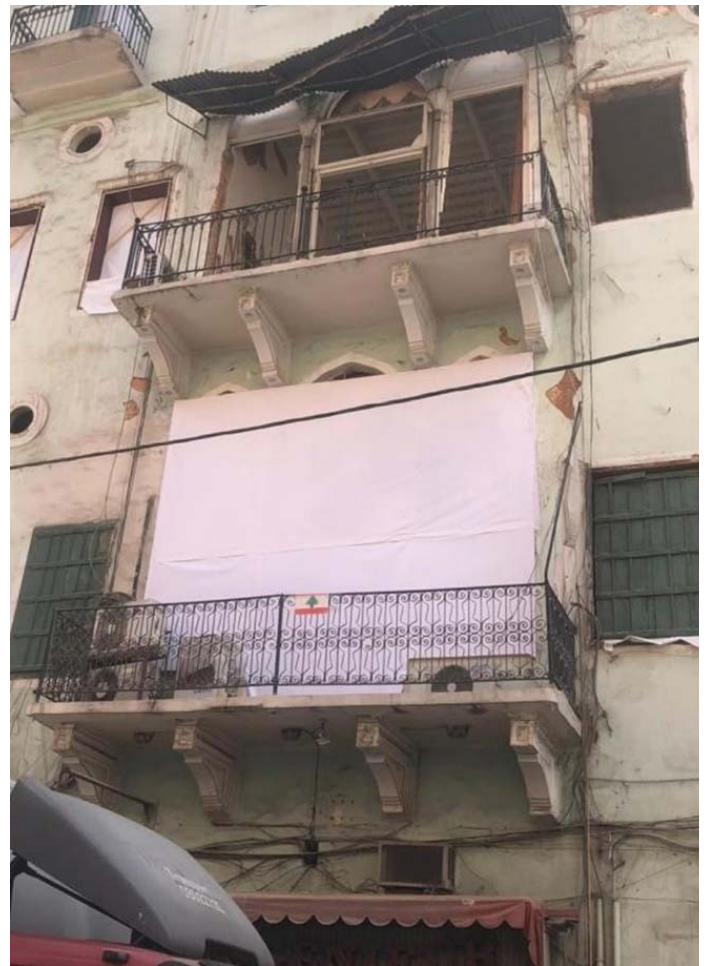
Ghoulam house A – plot 1137 Rmeil AFTER INTERVENTION
