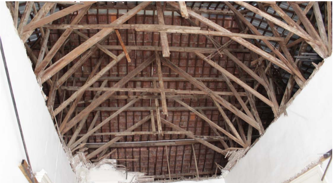
Roof covered and insulated from the elements
