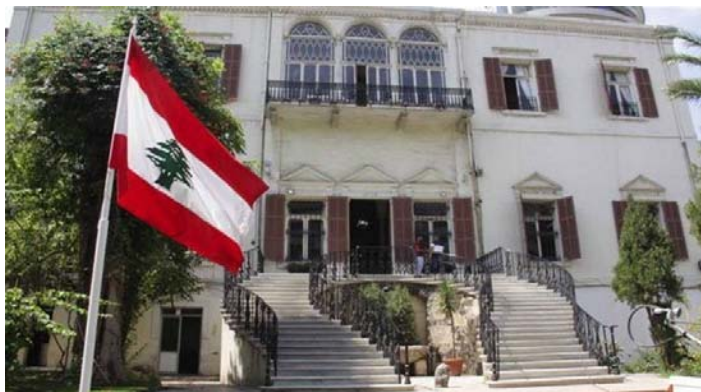
MoFA Building – plot 31 Rmeil BEFORE BLAST
