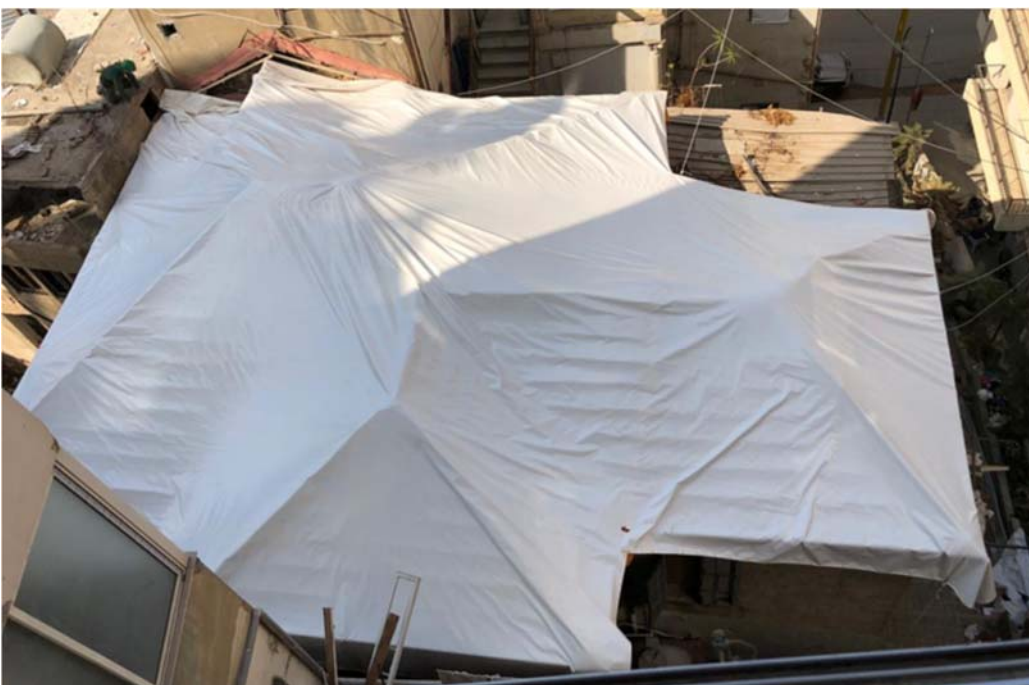
Ghoulam house B plot 474 Rmeil AFTER INTERVENTION
