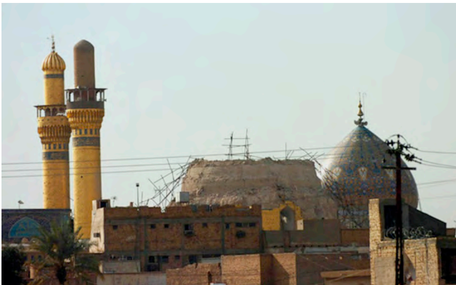
Figure 31.3 The extensive damage to the al-Askari Shrine in Samarra, Iraq in 2006 has been regarded by many as the tipping point that turned general unease with the coalition presence in Iraq into a full-scale, sectarian civil war. The minarets were destroyed in 2007. Image: PJF Military Collection / Alamy Stock Photo
